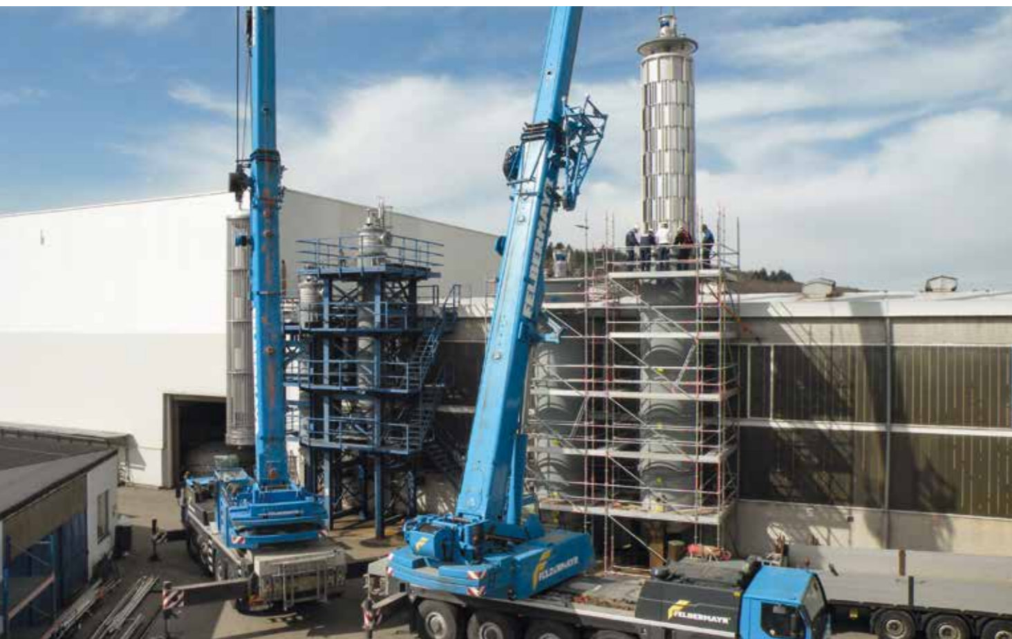
Installation of a short-path evaporator © GIG Karasek
