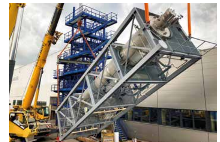
Thin-film evaporator – skid unit © GIG Karasek
